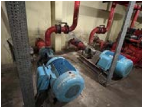
Figure: Centrifugal pumps
