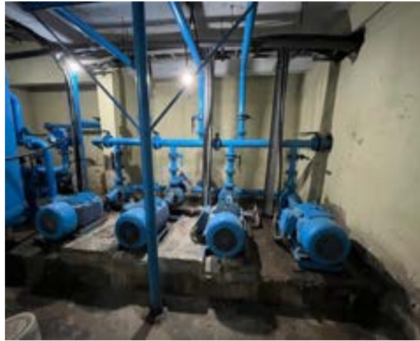
Figure: Pumps to overhead tanks
