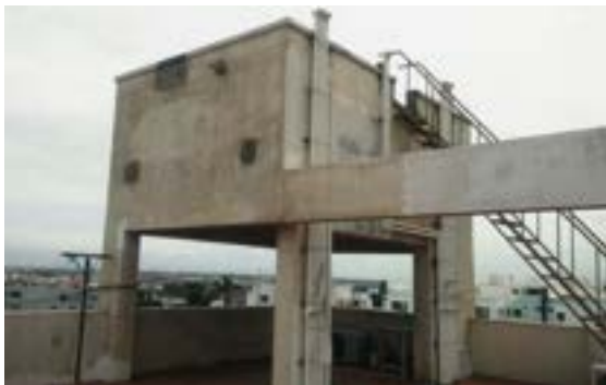
Figure: Overhead tank
