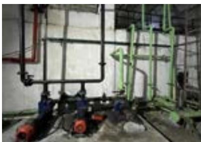
Figure: Sewage pumps to overhead tanks
