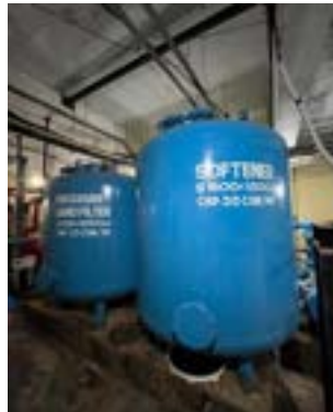
Figure: Water softener, pressure sand filter
